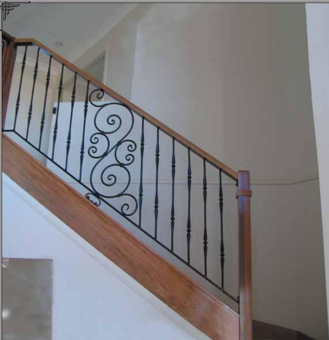
NB36-01 Wrought iron panels used with timber posts and timber top rail
